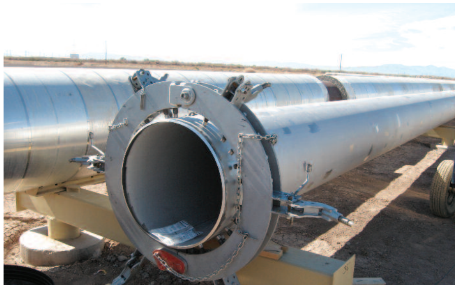
Heavy duty rim line-up clamps
