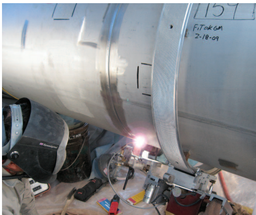
Carolina Energy Solutions orbital machine welding
